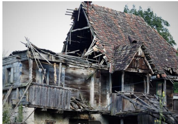
Figure 2: Dai stilted house destroyed by the earthquake
