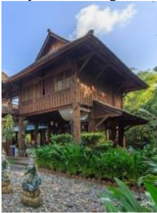
Figure 1: Dai stilted house
