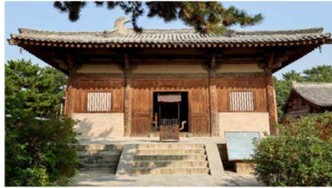
Fig.1 A photo of the front facade of the Main Hall of Nanchan Temple
