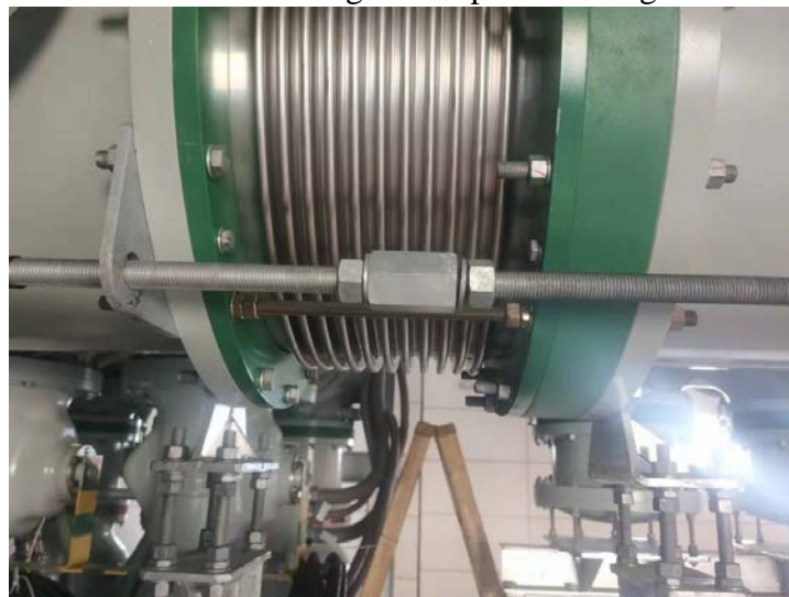
Figure 1: The bellows and the adjusting screw
