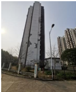
(a) Apartment Scan Overview
