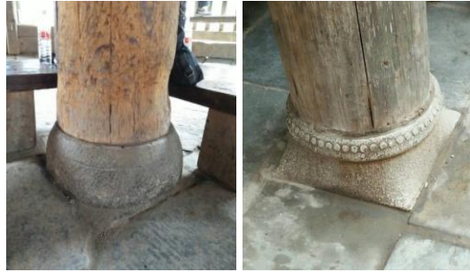
Figure 6: The connection between columns and column base stones
