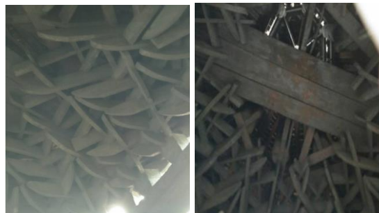
Figure 7: The connection between the tower top and the main body of the drum tower
