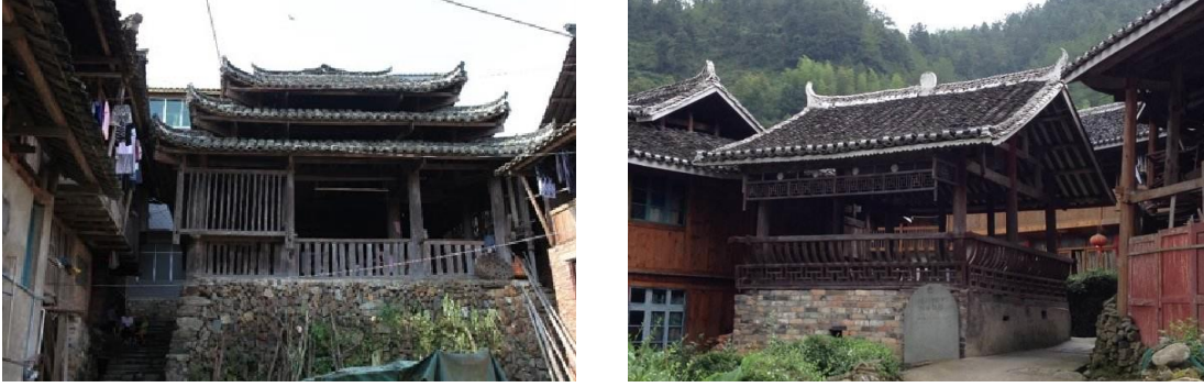
(a)The RHC style drum tower (the Jiang Bian drum tower in Pingzhai Village. (left) (b)The Overhanging roof column-and-tie-beam style drum tower. (right)
