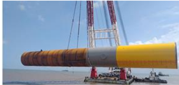
Figure 1: Monopile Foundation Structure
