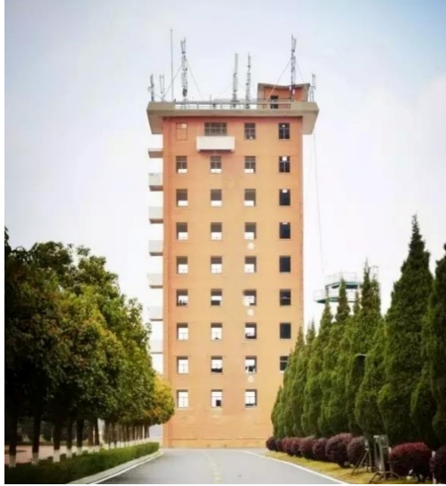
Figure 1. The existing Fire-fighting rope rescue training tower
